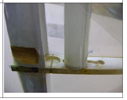
TO FILL THE HOLE WITH A CORK IN WOOD (IF IT IS NECESSARY)
